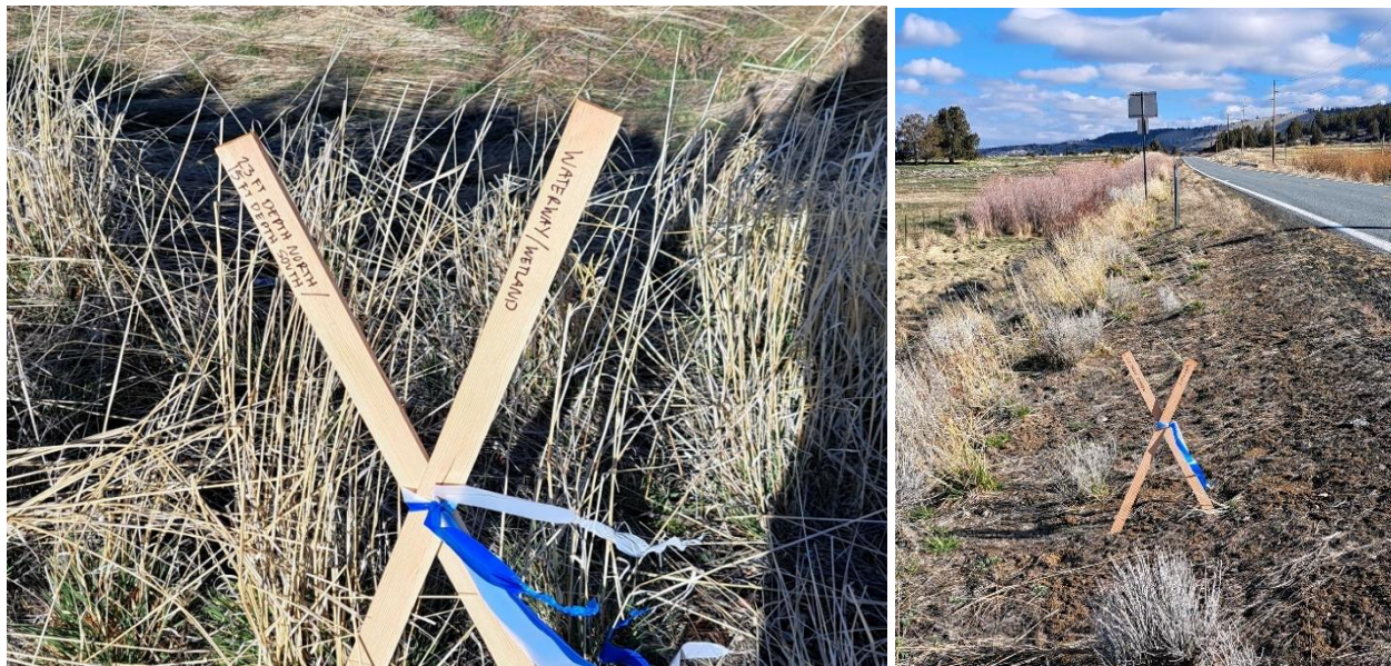
Photo 5 and Photo 6. Resource staking and flagging with bore depths (bore depths based on vegetation communities at crossings per AMMs). 50-foot setback from edge of resource built into exclusion areas.
