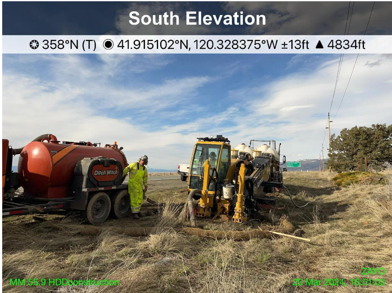
Photo 13: HDD equipment with straw wattle (BMP) and Vac-Truck.
