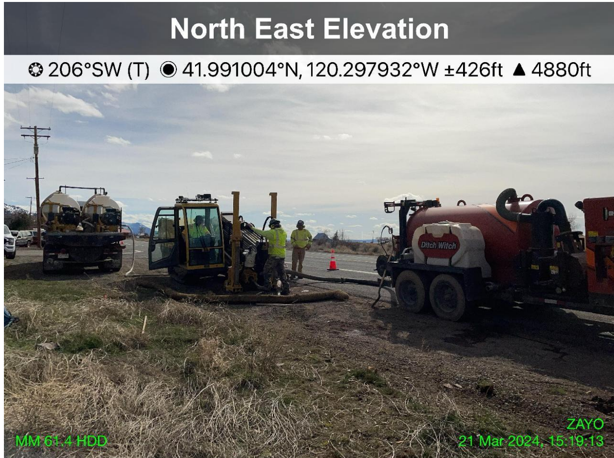
Photo 14: HDD equipment with straw waddle (BMP) and Vac-Truck.
