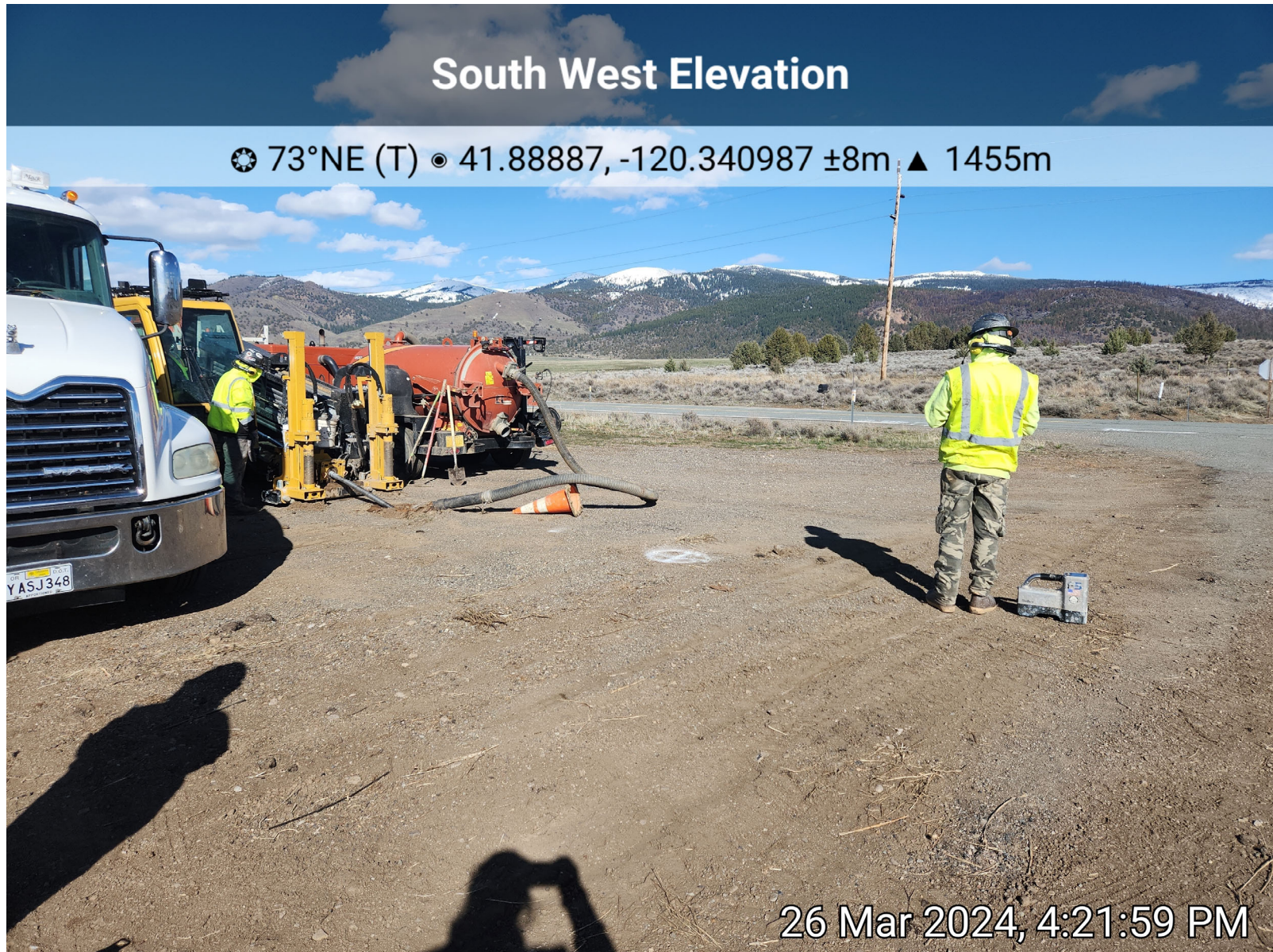
Photo 1: View of HDD at MP 54. The detector to the right shows approximate location of drill
